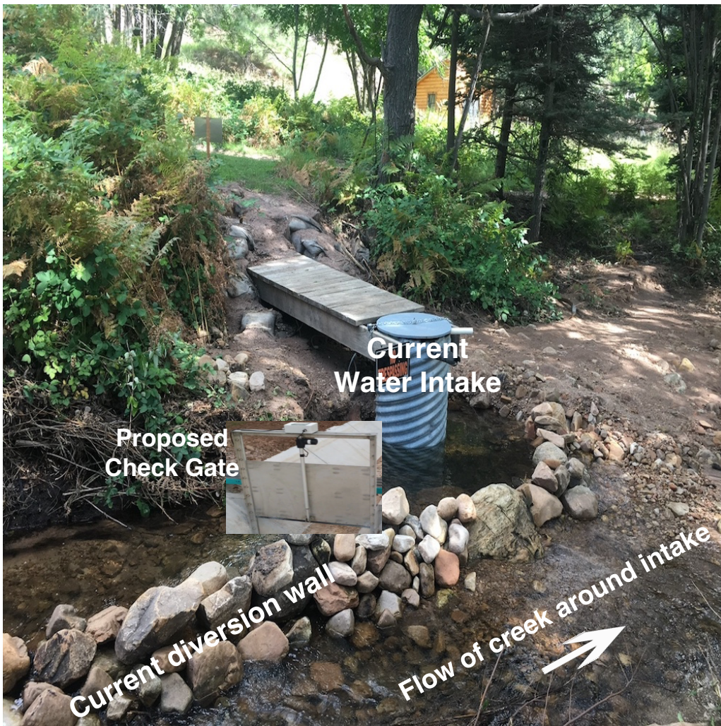
PHOTO OF CURRENT BONITA CREEK WATER COMPANY INTAKE
